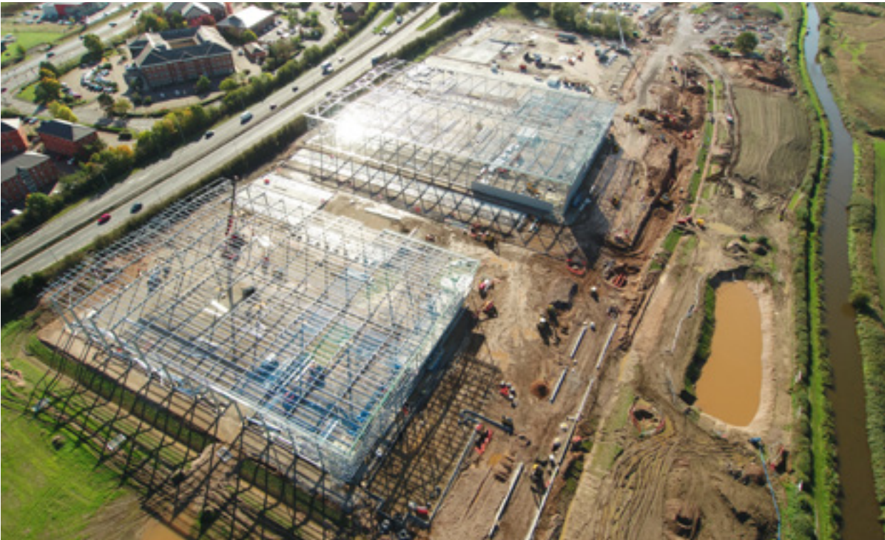
Quintus, Burton, Derbyshire – Adstone Construction Ltd
