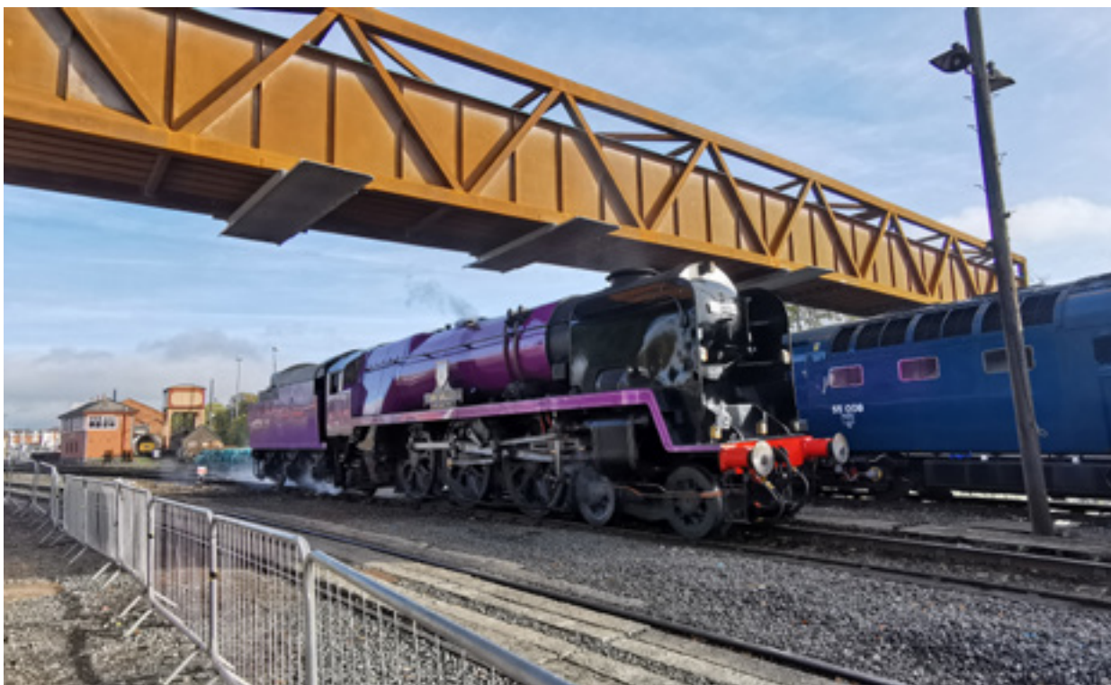
Severn Valley – Heritage Rail, Kidderminster Station – Adey Steel Ltd
