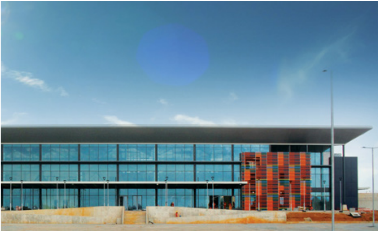
Airport Terminal, Kumasi, Ghana - REIDsteel
