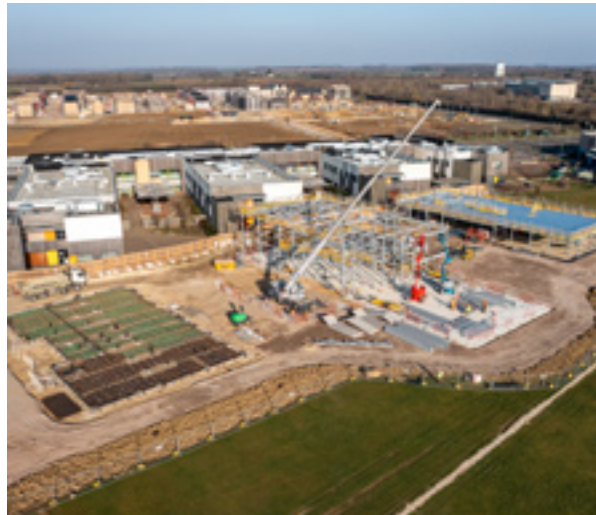
Cambourne Secondary School, Cambourne – SDM Fabrication Ltd
