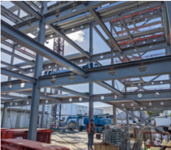
Studio 5, Power Road Studios, Chiswick, London – TSI Structures Ltd
