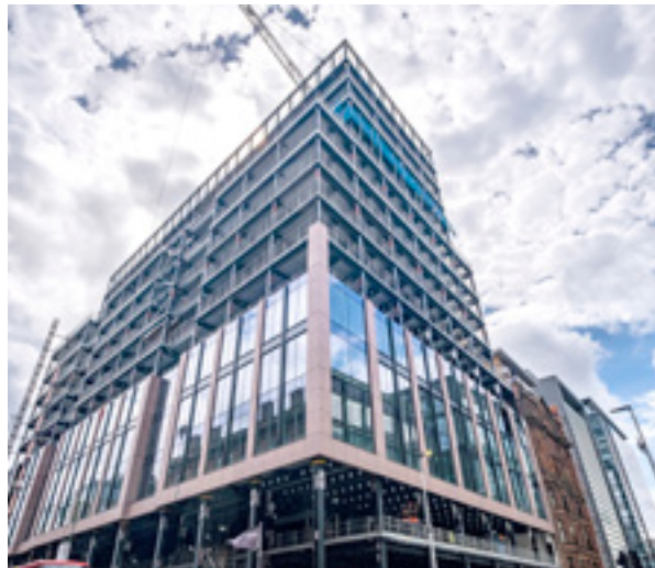
Argyle Street, Glasgow - Severfield plc
