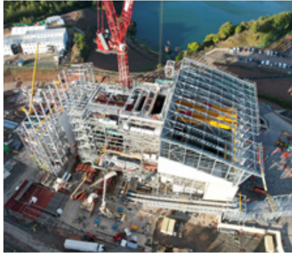
Sandwell Aquatics Centre, Birmingham – Billington Structures Ltd
