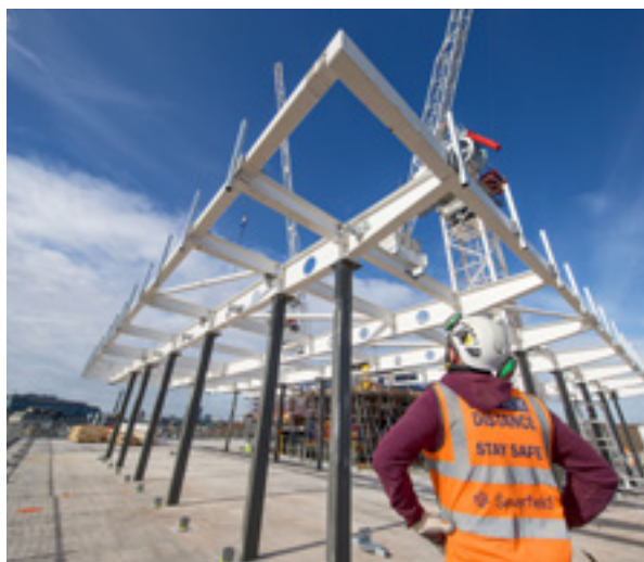
150 Holborn, London – Severfield plc
