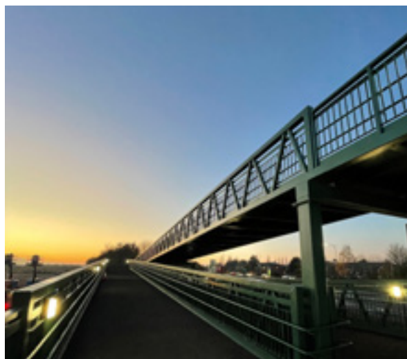
Church Lane Bridge, A45, Solihull, Birmingham – Skanska Fabrications
